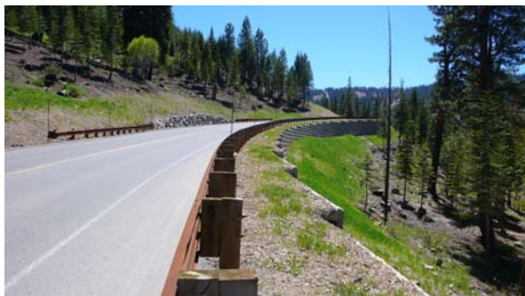
Treated cut and fill slopes along Highlands View Road, one year following treatment
