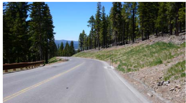
Treated cut and fill slopes along Highlands View Road, one year following treatment
