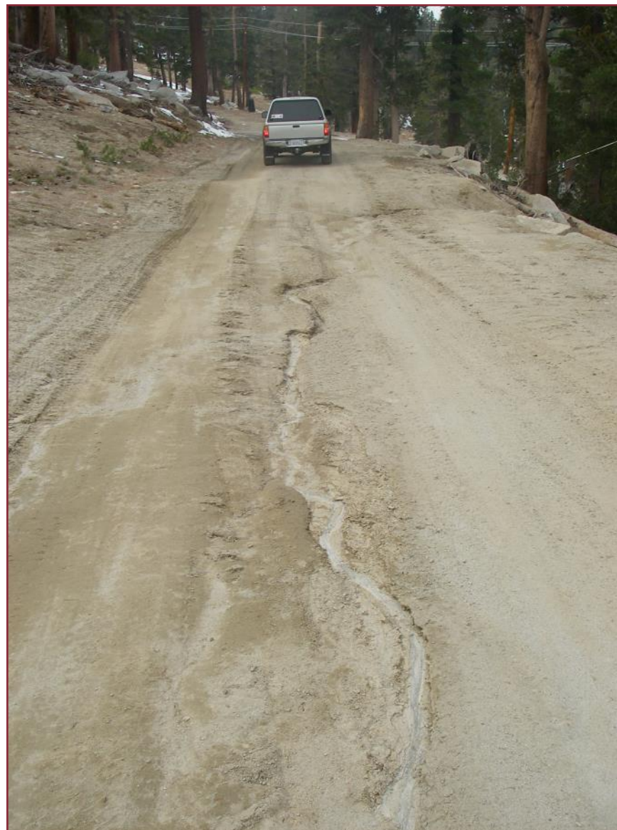
The road is insloped, yet water has formed a rill down the center of the road and is down-cutting at the rolling dip.
