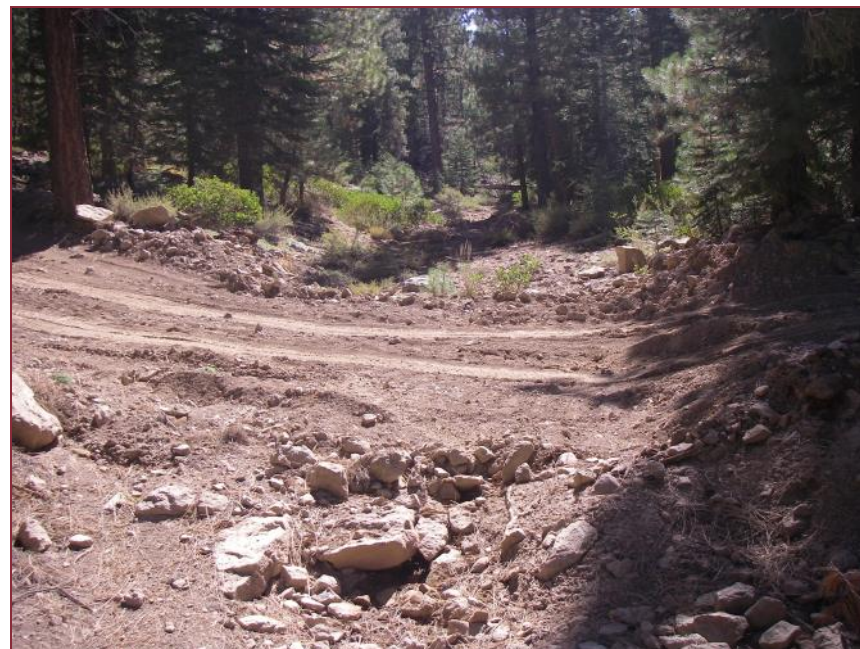
A recently graded logging road intersects with an ephemeral drainage near Truckee, CA. Sediment from this roadway is directly connected to this drainage, which has high connectivity to a Lake 500 feet downstream. This is one of many examples of the interconnected nature of erosion issues in high-use watersheds.
