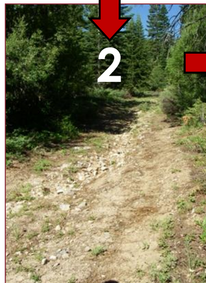
Confirmation of road flow capture and erosion in field.
