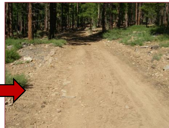
Truckee Haul Road – one season after smooth grading, rilling was observed in the exact same location as the gully.
