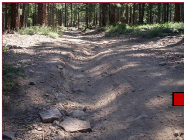
Truckee Haul Road – large gully present before smooth grading.
