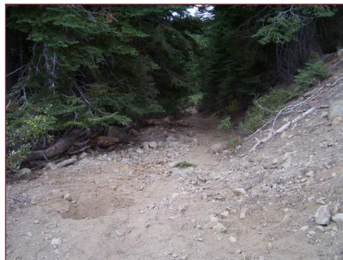
Lower Lombard Road before treatment with compacted, bare soil.
