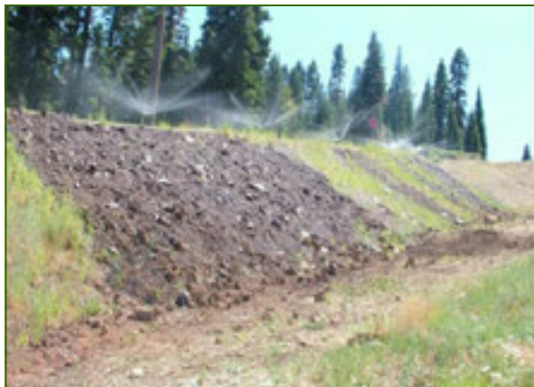
Northstar Superpipe – failure caused by over-irrigation (left); repaired slopes with proper irrigation (center); stabilized slopes two years after treatment (right).
