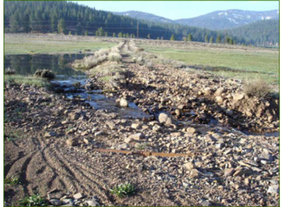
An obvious erosion hot spot on a road segment in the Martis Valley where meadow drainage was not accommodated.
