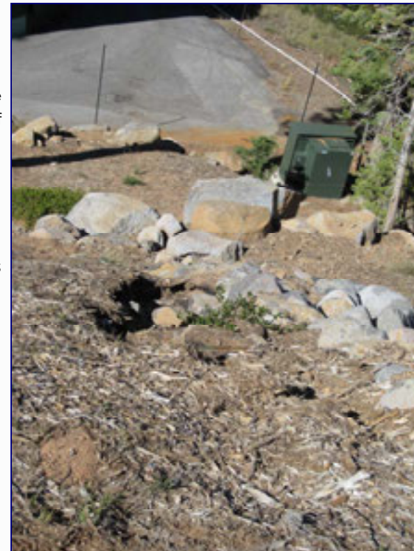
A gully on this slope indicates active erosion, which is the need for action at this site.
