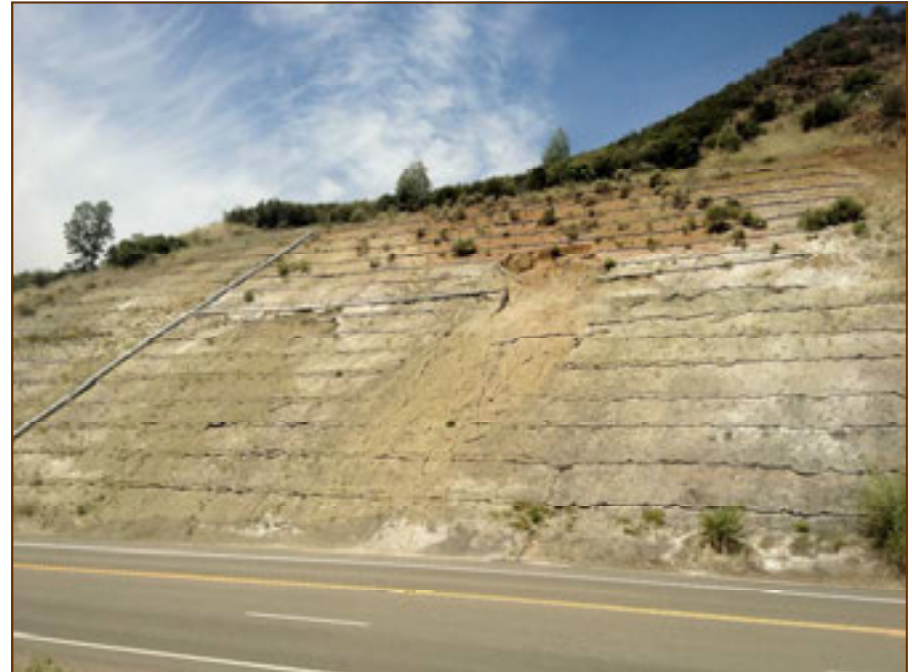
This compacted road cut slope exhibits widespread erosion and a slope failure, largely due to lack of infiltration capacity.
