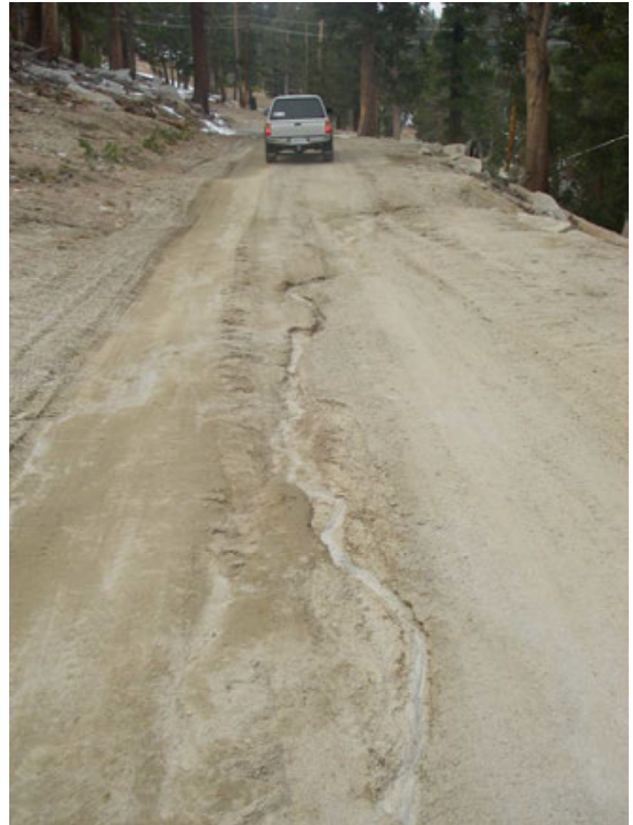
The road is insloped, yet water has formed a rill down the center of the road and is down-cutting at the rolling dip.
