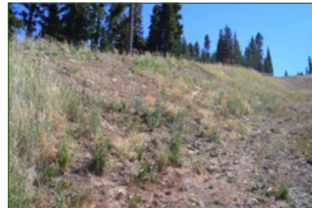
Northstar Superpipe – failure caused by over-irrigation (left); repaired slopes with proper irrigation (center); stabilized slopes two years after treatment (right).
