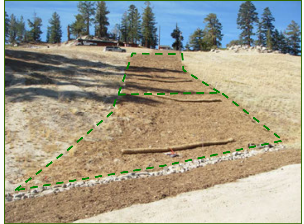
Test plots were integrated into this post-construction restoration treatment following installation of a waterline at Heavenly. The treatment area was simply divided in half and two different soil amendments were used. Photo taken one week after treatment.
