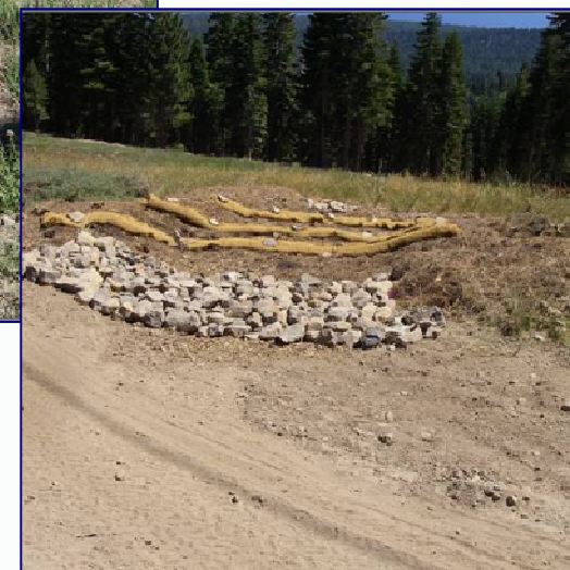
Example of installing an infiltration swale to prevent road runoff from causing erosion further downslope.
