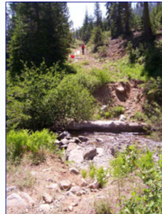
Severe erosion at abandoned road-stream crossing.
