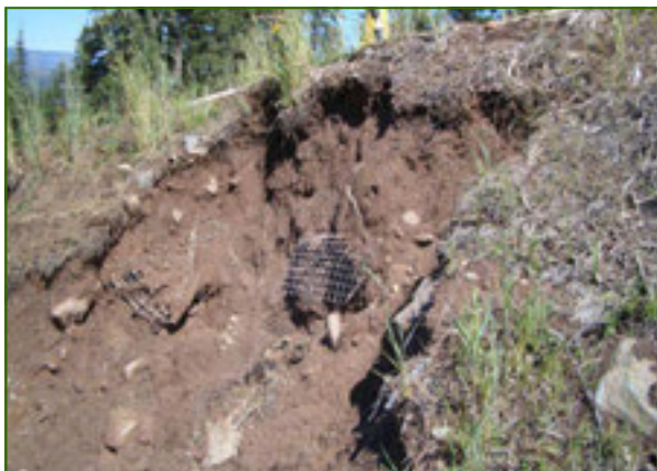
Northstar Superpipe – failure caused by over-irrigation (left); repaired slopes with proper irrigation (center); stabilized slopes two years after treatment (right).
